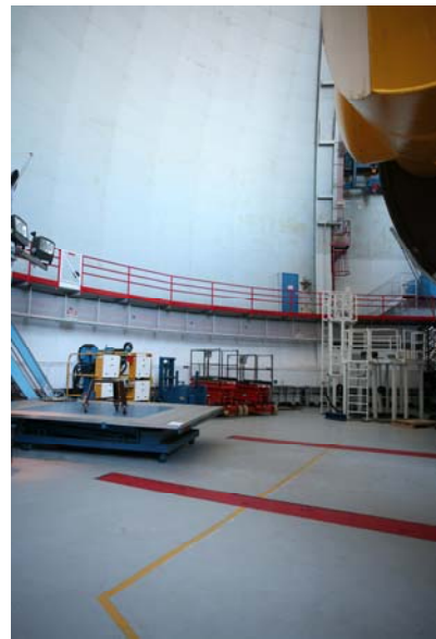
Vent apertures should not extend below the top of the blue doors at the catwalk level in order to avoid electrical supply boxes and other obstructions.
