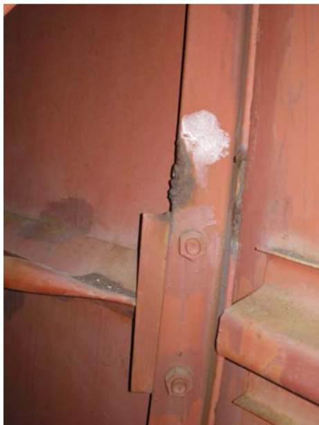
Figure 8, 9 and 10 Further details of rib bracing web frames
